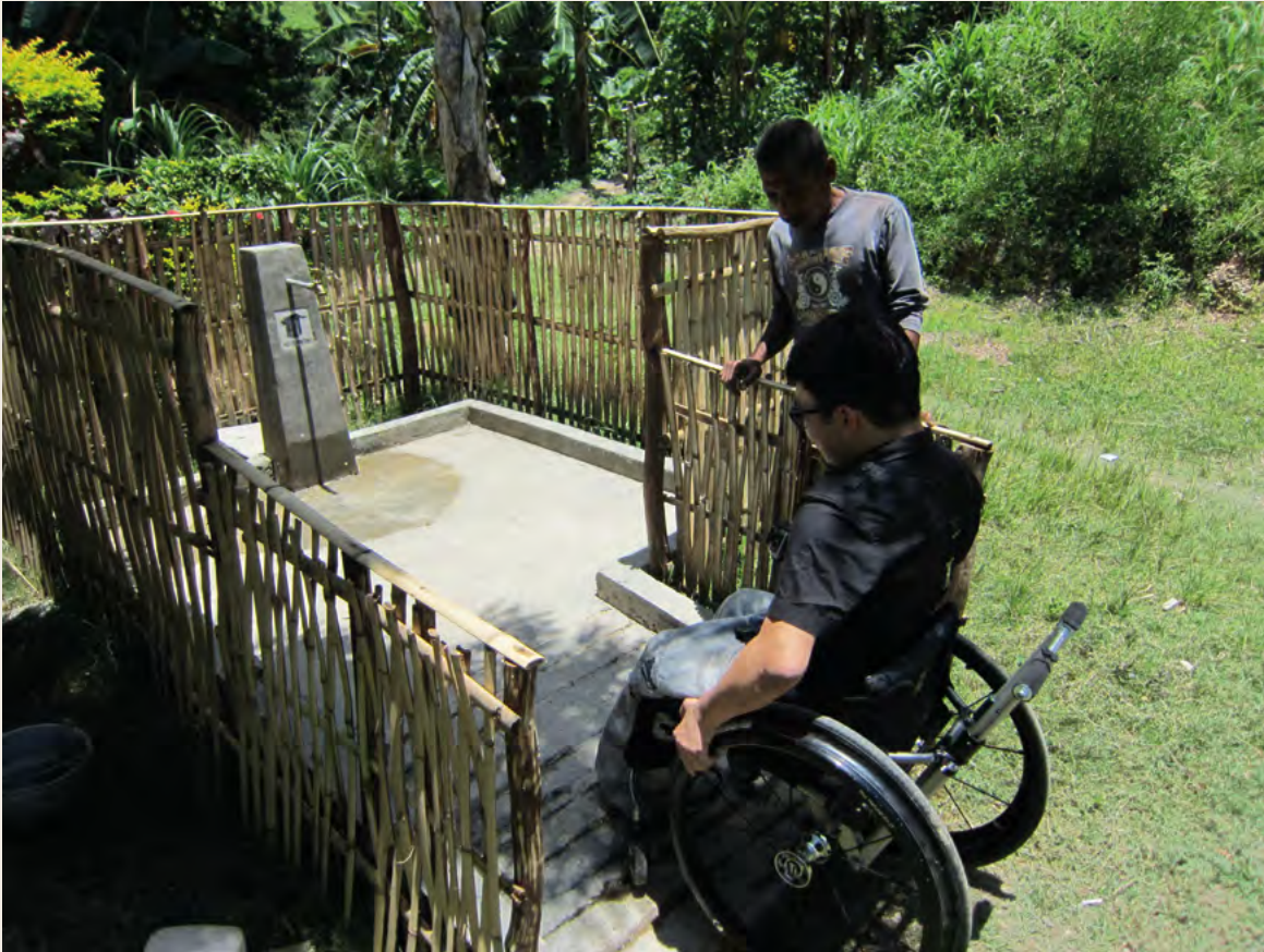
WaterAid Australia Equity and Inclusion Officer trialing the new water point access in the Aldea. © WaterAid Timor-Leste
