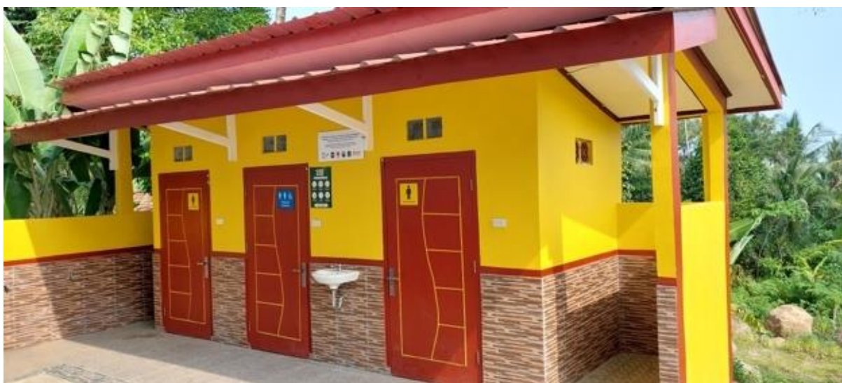
An example of accessible sanitation and evacuation facilities done by ASB in Indonesia. © ASB
