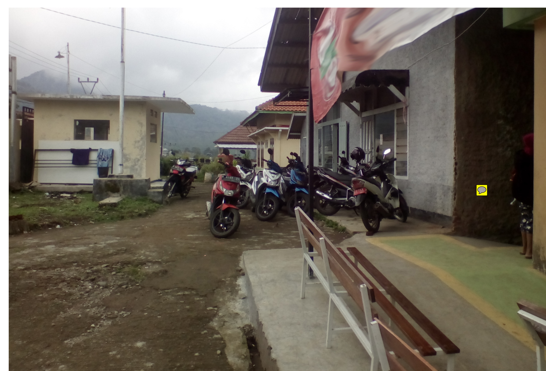
Figure 2: Ramp obstructed with motorbikes and benches in a primary health center
