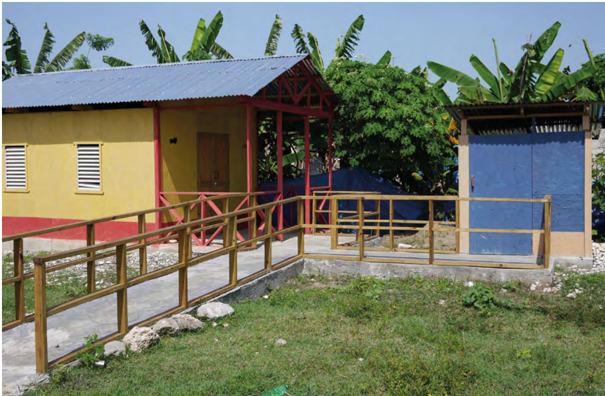
Accessible path between shelter and sanitary facilities (example from Haiti). ©CBM and Help e.V, Haiti
