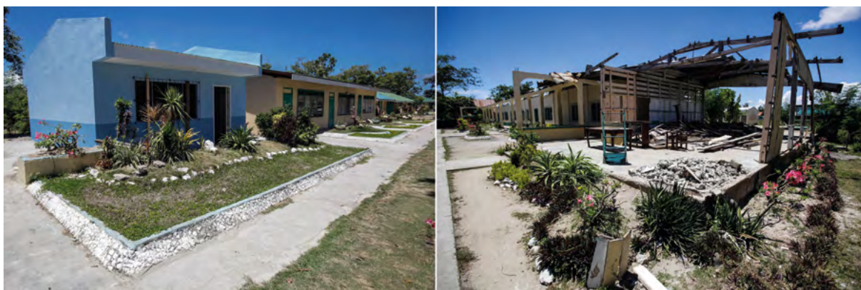
New resource centre for Carles School in Iloilo (left), and the old building (right), which was completely destroyed by typhoon Haiyan.
